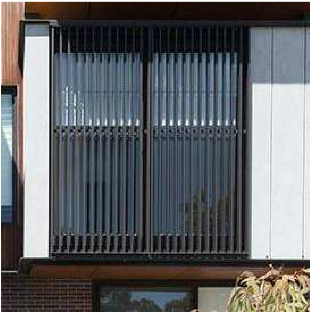
7. ALUMINIUM LOUVRES - ELLIPSOID BLADES
