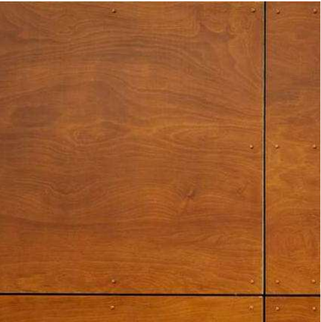
5. EXTERNAL PLYWOOD SOFFIT
