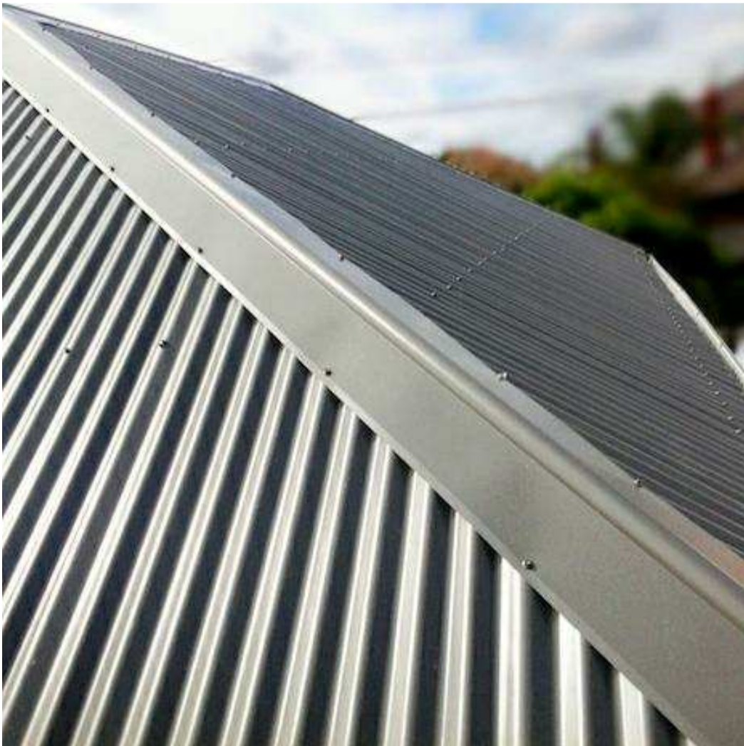
4. BLUESCOPE ZINCALUME ROOFING - SPANDEK PROFILE
